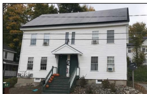
Behind-the-meter solar installed on Avery Hill multifamily rental housing buildings.
