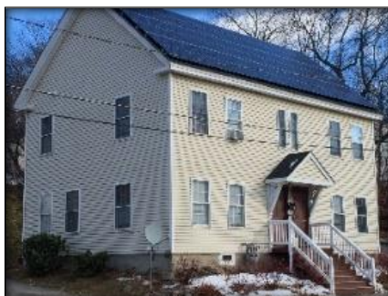
Behind-the-meter solar installed on Avery Hill multifamily rental housing buildings.
