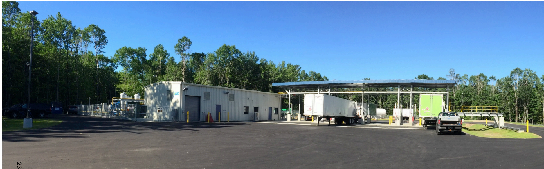
CNG Supply Terminal, Eliot ME – PNGTS and M&NE Joint Facilities
