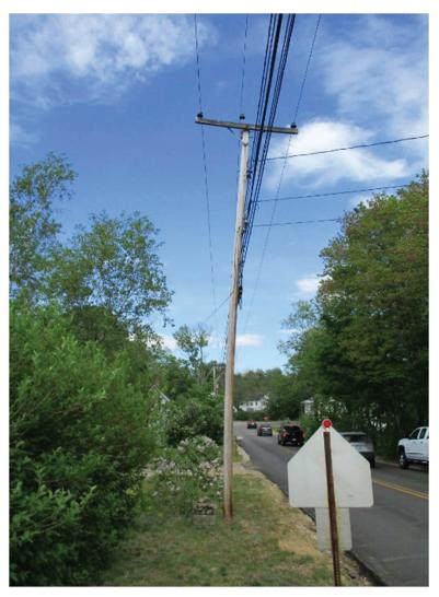
Figure 4-5. Structurally Overloaded Eversource Class 4 Wood Distribution Pole
