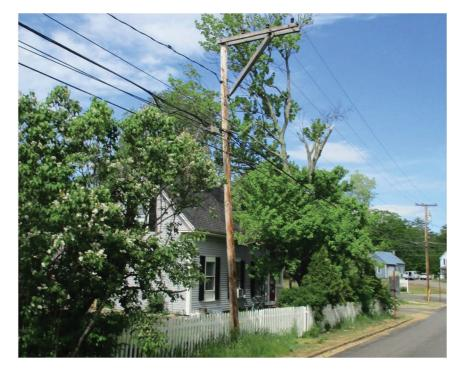
Figure 4-6. Structurally Overloaded 80+ year-old Eversource Wood Distribution Pole
