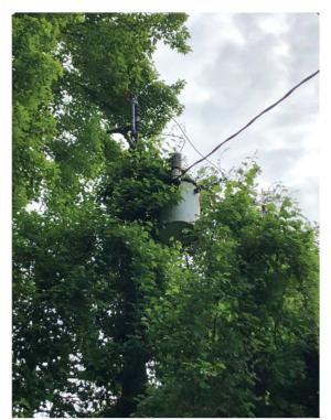
Figure 5-24. Vegetation on Distribution Transformer Pole
