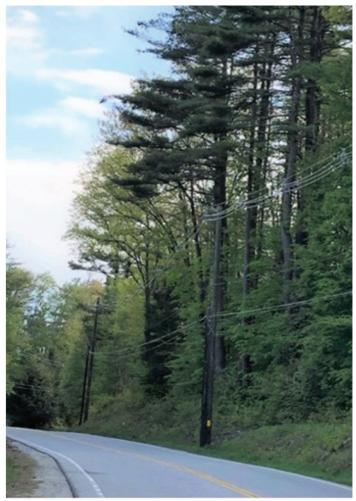
Figure 5-52. Eversource Line Reconductored to Spacer Cable
