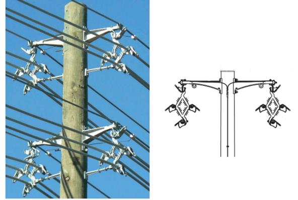
Figure 5-13. Image and graphic of spacer cable design showing compact nature of installations
