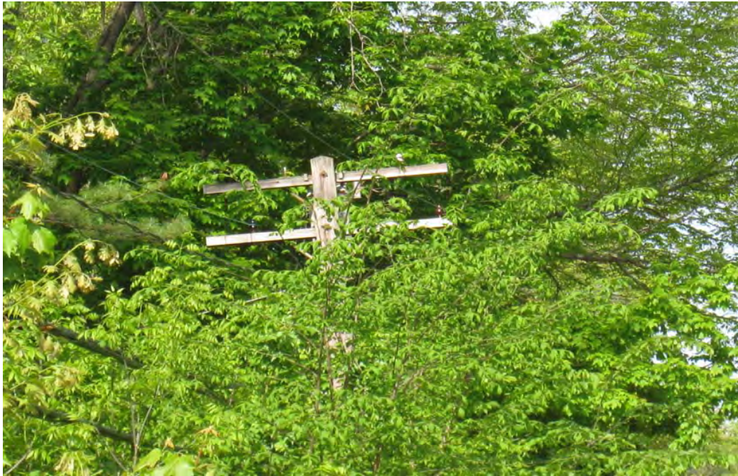
Figure V-14 – NESC Rule 218 violation in Until service area.
