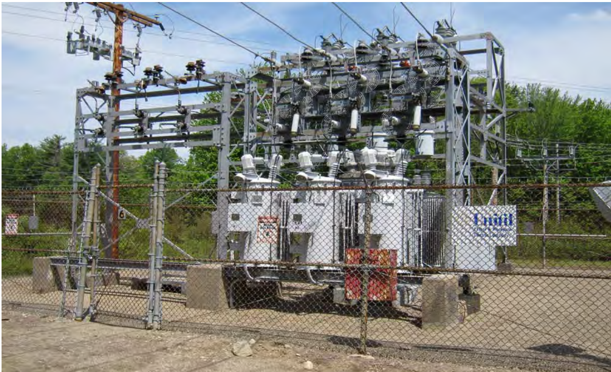
Figure IV-6 – 34.5kV to 13.8kV Unitil electric distribution substation located in East Kingston, New Hampshire. (Photo by NEI-Unitil System)
