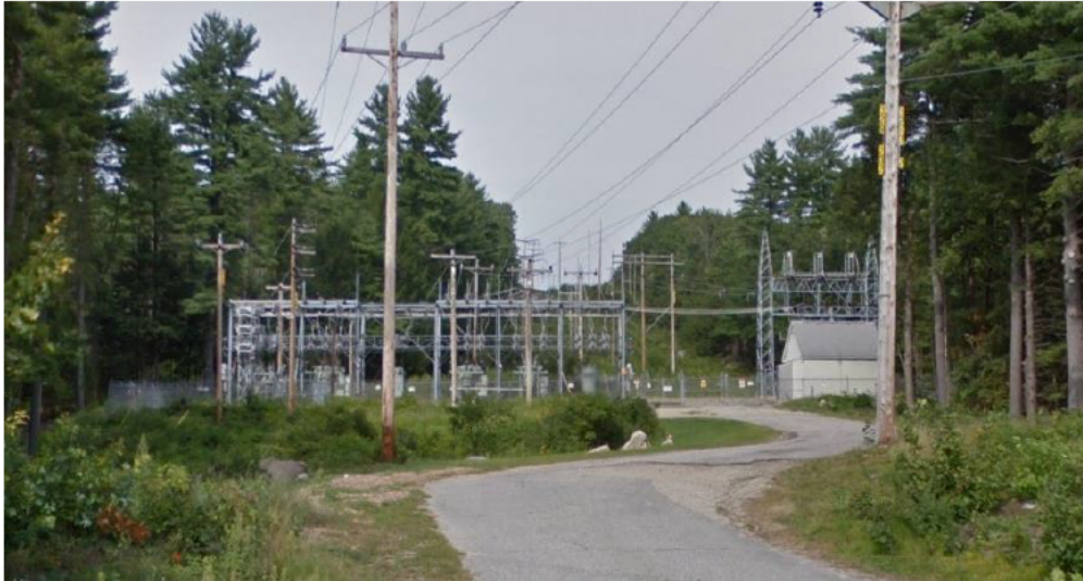
Figure 1. South Milford Substation viewed from Hammond Road, Milford.
