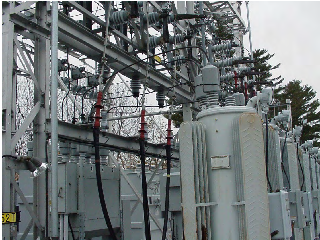
18L1 Regulators and relationship to cables
