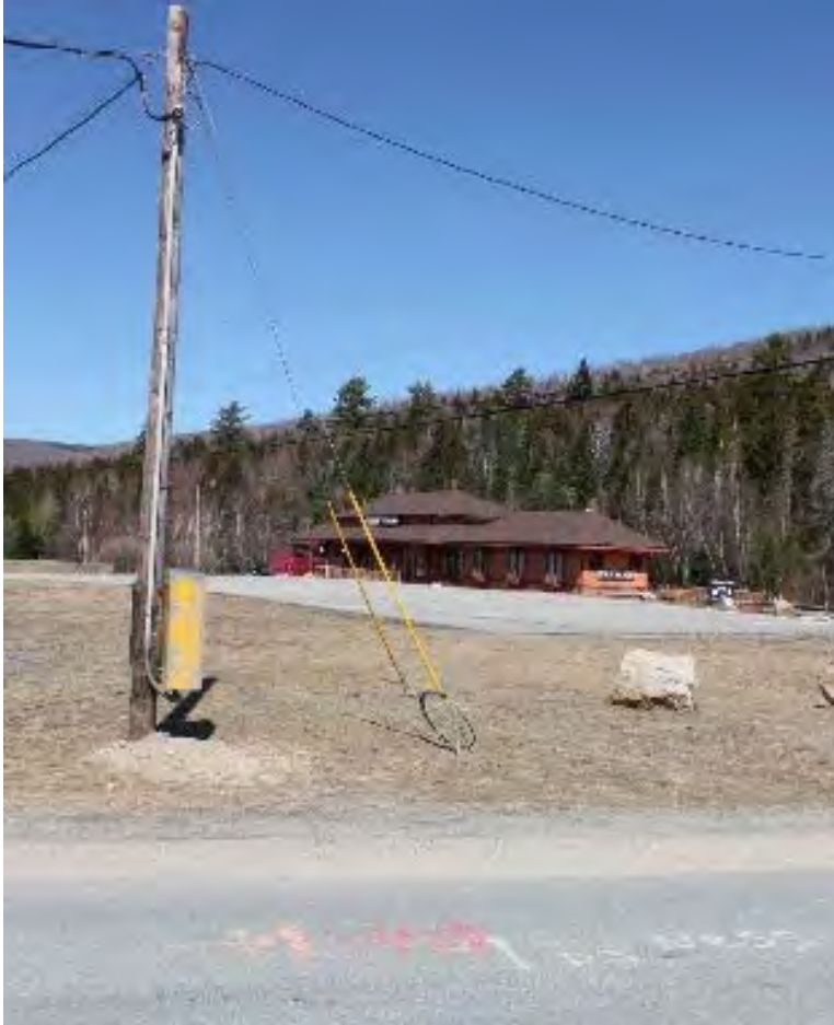
Photo 2-2 indicates an area in which excavation was performed but no markings by AWC are shown. Puc 800 rules require markings of any underground water mains within established tolerance zones or provide positive response that no water mains are present within the tolerance zone.
