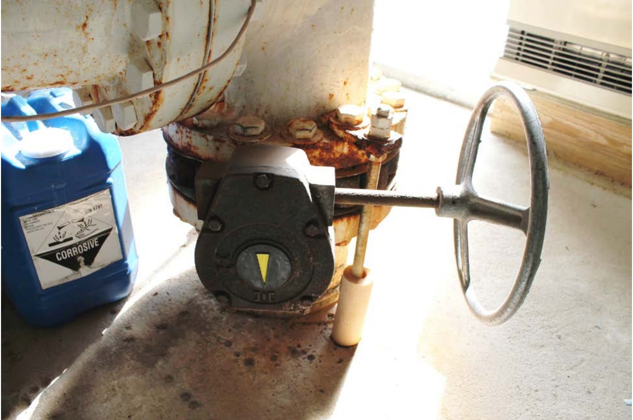
Photo #5-02 Depicts main system shut off valve noting storage of corrosive chemicals.
