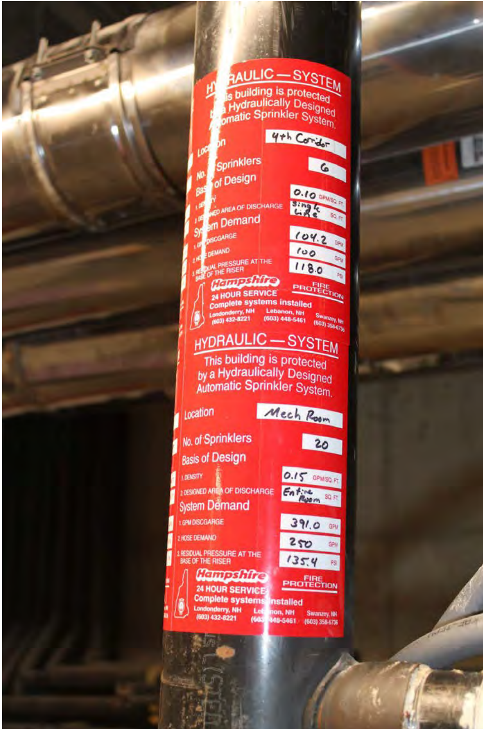
Photo #5-05 View of hydraulic data plates on Mt. Washington hotel fire protection, noting a system demand of 135 psi.
