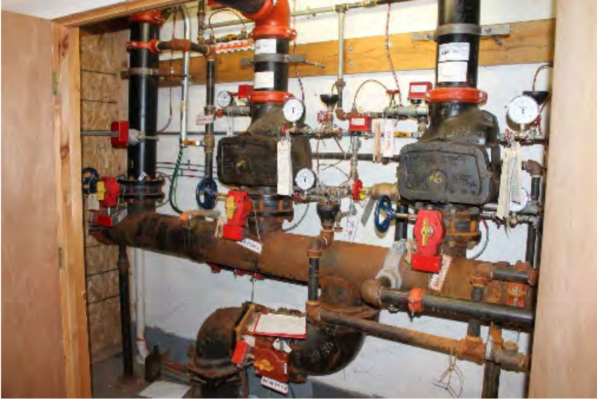
Photo #5-03 View of several fire sprinkler system risers at Mt. Washington Hotel.
