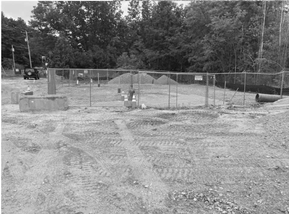
Completed Base of Regulator Station
