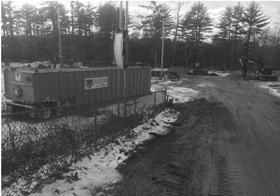
Exit Pit Container
