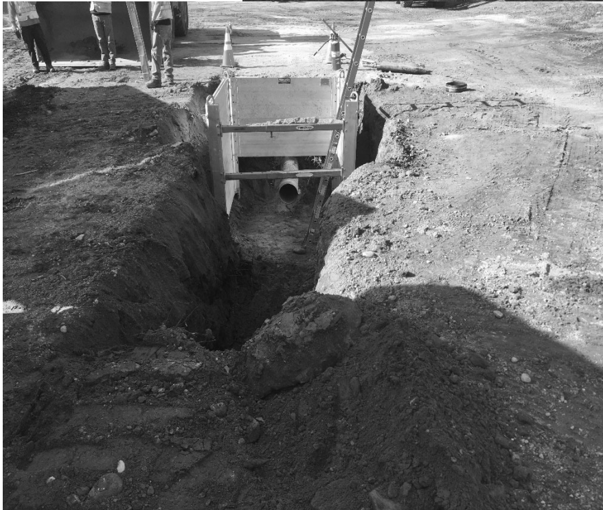
View of Pipe in Trench
