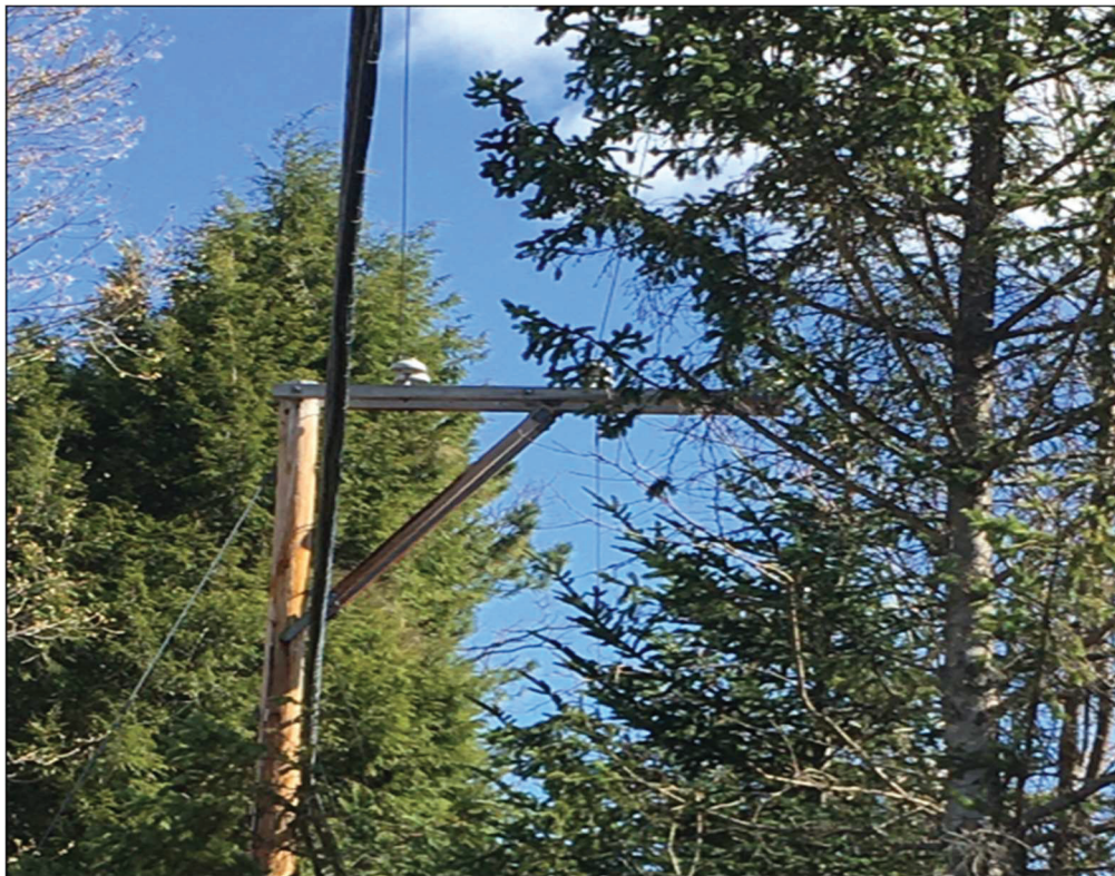
Source: TRC Field Inspection
