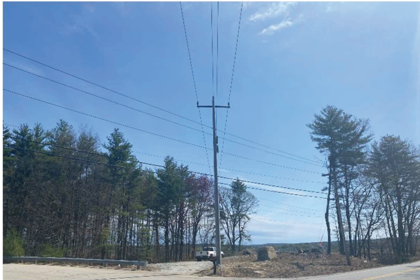
Figure 5-33. Eversource circuit after ROW clearing
