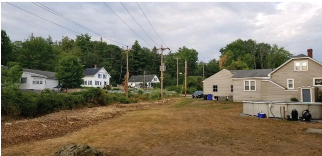
Figure 5-31. Eversource Circuit following ROW clearing
