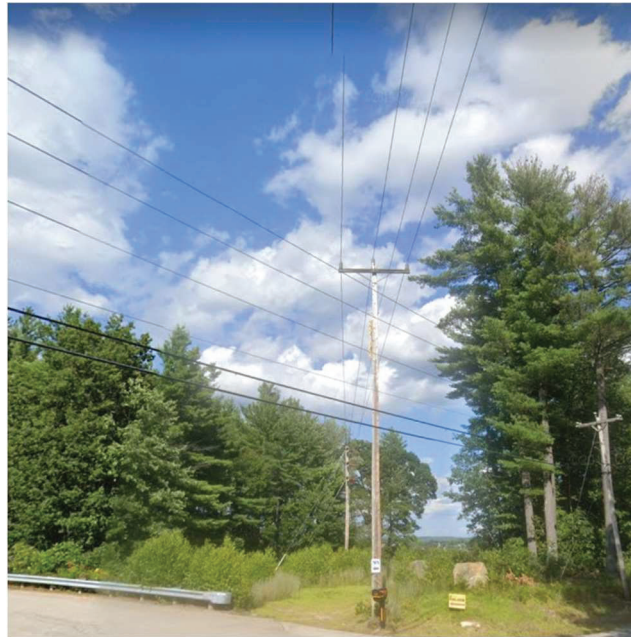
Figure 5-32. Eversource circuit prior to ROW clearing
