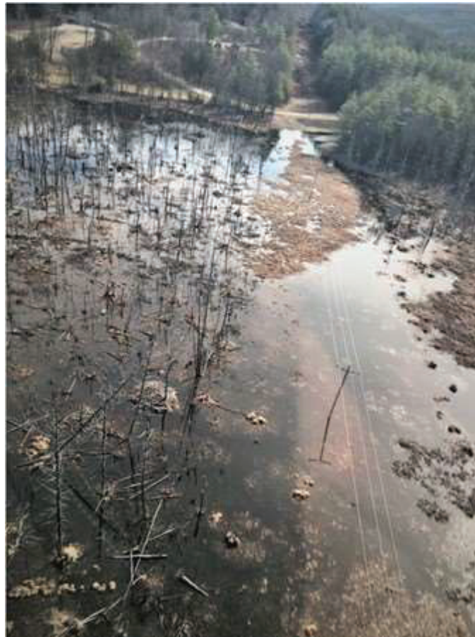
Figure 5-50. Eversource Line 317 Line Relocation
