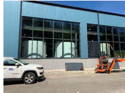
Storefront glass at chemical storage areas, such as the example in this photograph, has the functional benefit of visual connection from the outside. This can aid operations personnel in detecting bulk loading over-fill or other anomalies from the outside.
