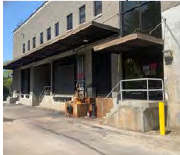
Maintaining access to chemical fill stations and loading dock is critical
