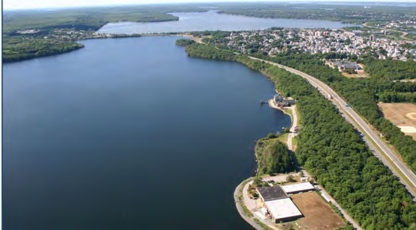
Water Treatment Plant at North Watuppa Pond
