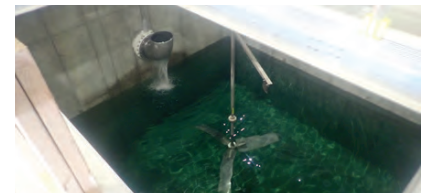
Flocculation basin hydrostatic testing.
