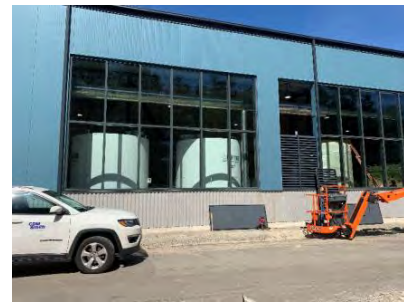
Storefront glass at chemical storage areas, such as the example in this photograph, has the functional benefit of visual connection from the outside. This can aid operations personnel in detecting bulk loading over-fill or other anomalies from the outside.
