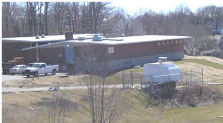
Babson Water Treatment Plant
