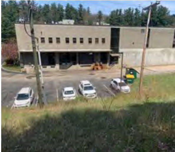
Potential location of new chemical storage
