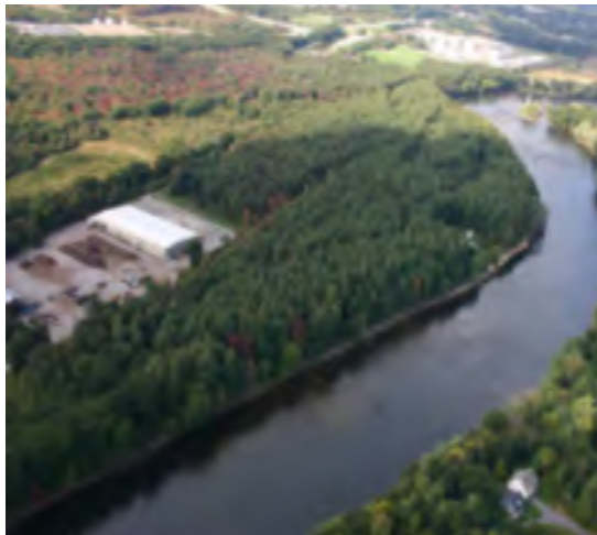
Merrimack River Intake
